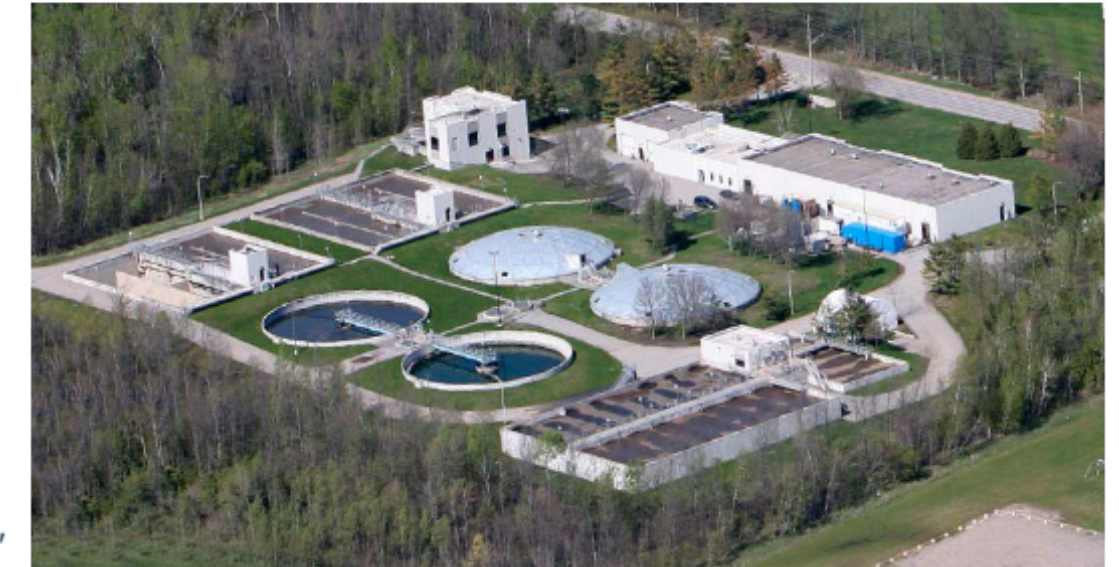
Wastewater Treatment Plant - 1578 St. John's Road
